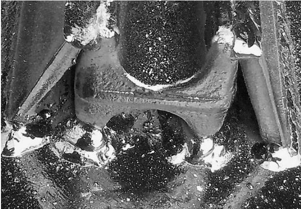
Figure 16: Example of poor installation
